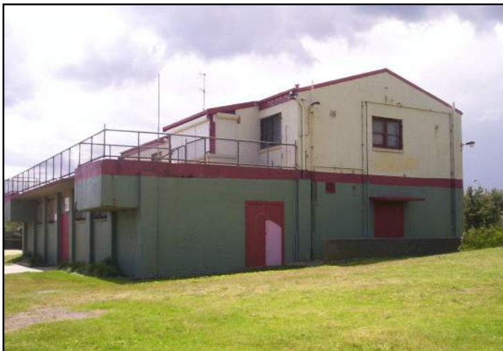
The Mordialloc Life Saving Club rooms – from 1957, it was home to various incarnations of the Shindig dance—making it one of the earliest rock 'n roll venues operating in the suburbs. The bottom section was for storage and the top floor hosted the dance action.
