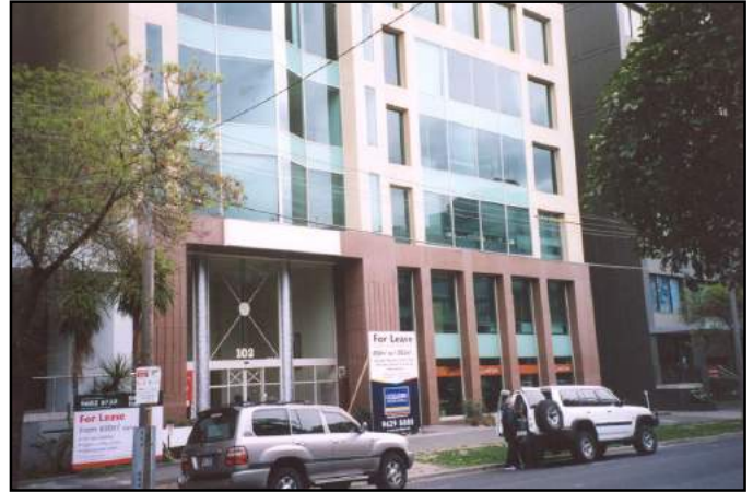
Progress in Albert Road, South Melbourne has ensured that multi-storied buildings now occupy the places where Bill Armstrong's single- and double-story Victorian terraces, once stood.
