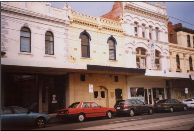
The Fortress-like entrance to what was Garrison Discotheque in High Street Prahran is still evident in the building which is remarkably intact and probably much as it was. The shield to the right of the doors can be clearly seen – it carried the logo used by Madder Lake.
