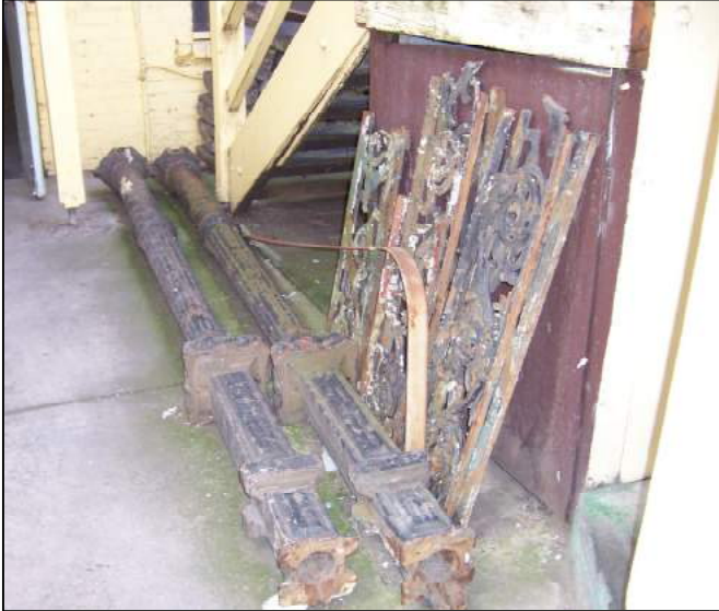
These cast iron posts once were located right smack-bang in the centre of the ground floor at Garrison. How many dancers bumped into them during a set by Madder Lake, Chain or The La De Das?
